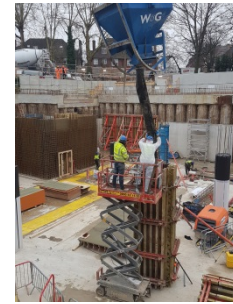
Casting of concrete columns
