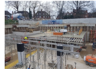
Falsework being erected for level 01 slab
