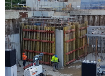
Core wall construction
