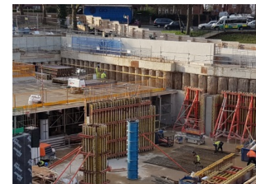
Decking being erected for level 01 slab
