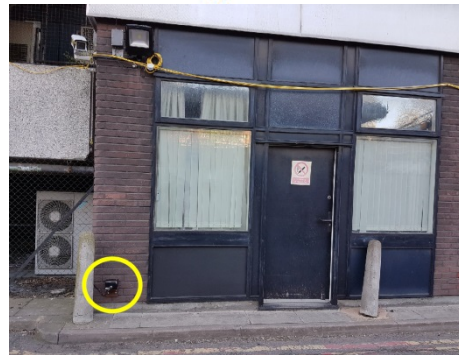
MRI Scanner Room 4
