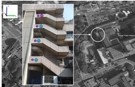
North-West External Concrete Stair
