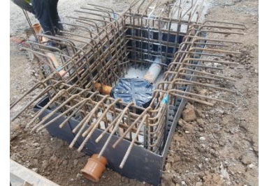
Underslab drainage
