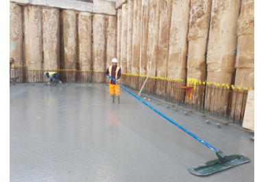
Casting of Basement Slab
